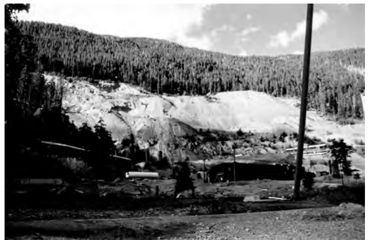
FIGURE 3.3-3b. Photograph of a Type 3 Mined-Rock Pile (by K.A. Morin).
