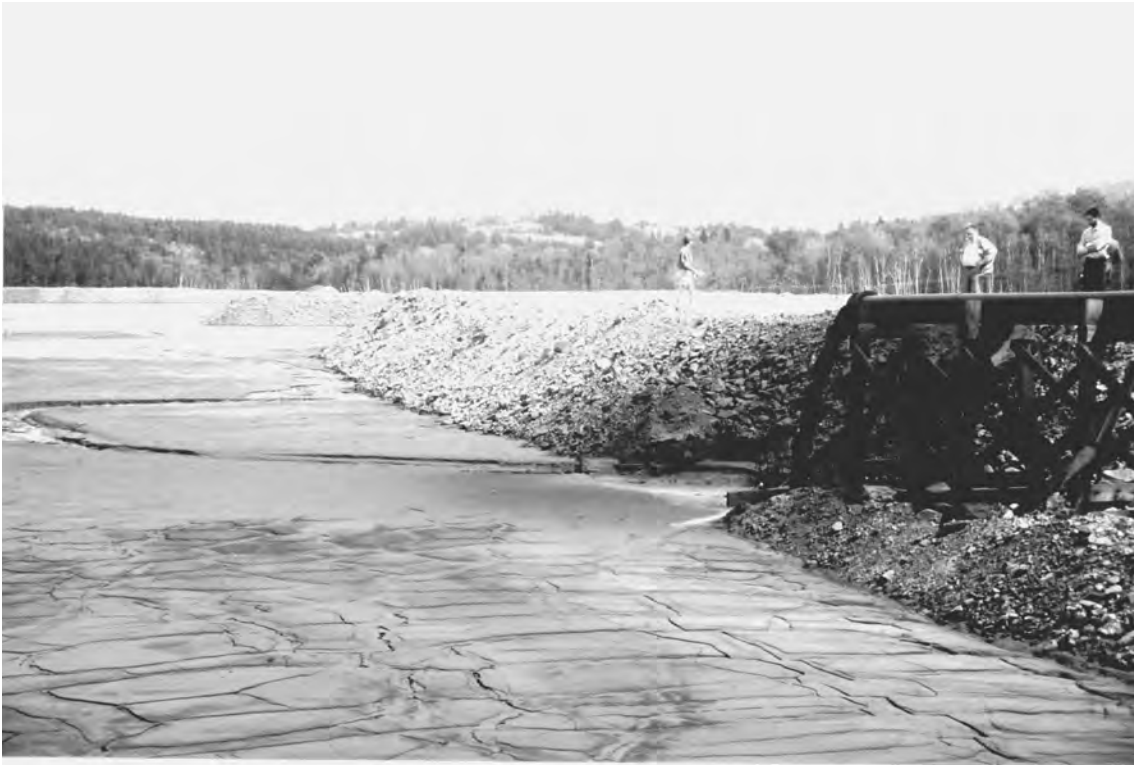
Tailings Impoundment; note active discharge pipe on right.
