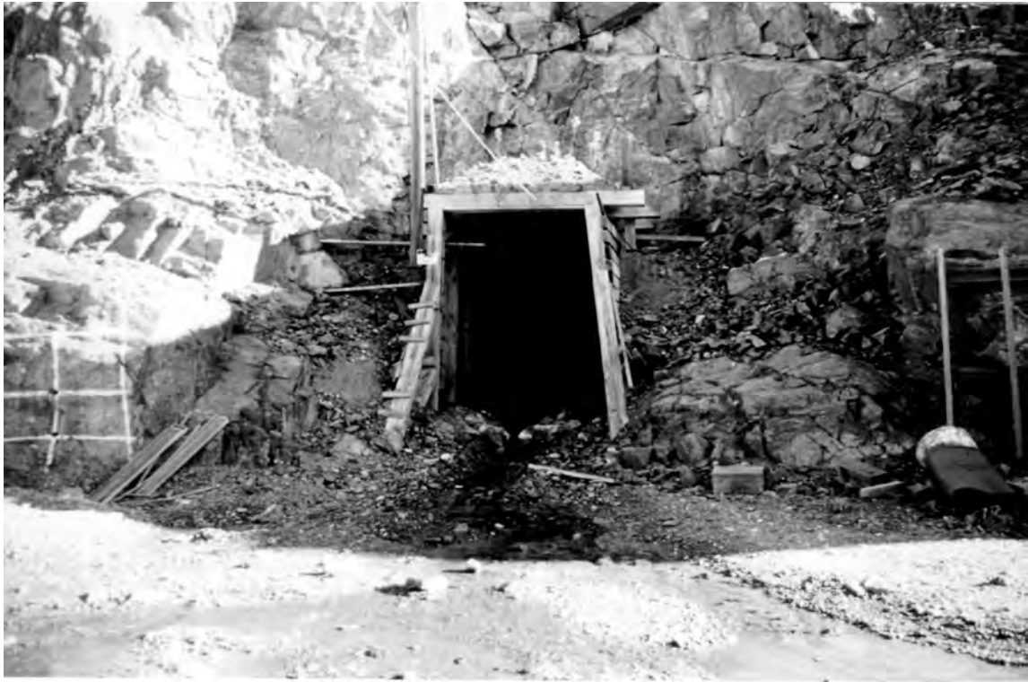
Looking at the Portal to a Type 2 Underground Mine; note gravity drainage.
